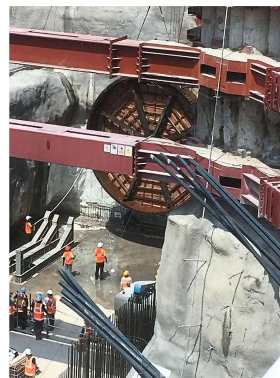
Shuttering pipe has been installed at Bandar Malaysia North in preparation for the launch of the first Tunnel Boring Machine.
