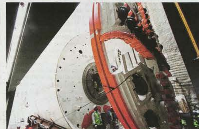
The cutterhead, part of the Variable Density Tunnel Boring Machine's components were lowered down to the shaft with extreme precision to ensure it fits to its other components
