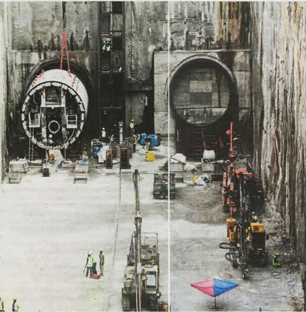
The cutterhead, part of the Variable Density Tunnel Boring Machine's components were lowered down to the shaft with extreme precision to ensure it fits to its other components
